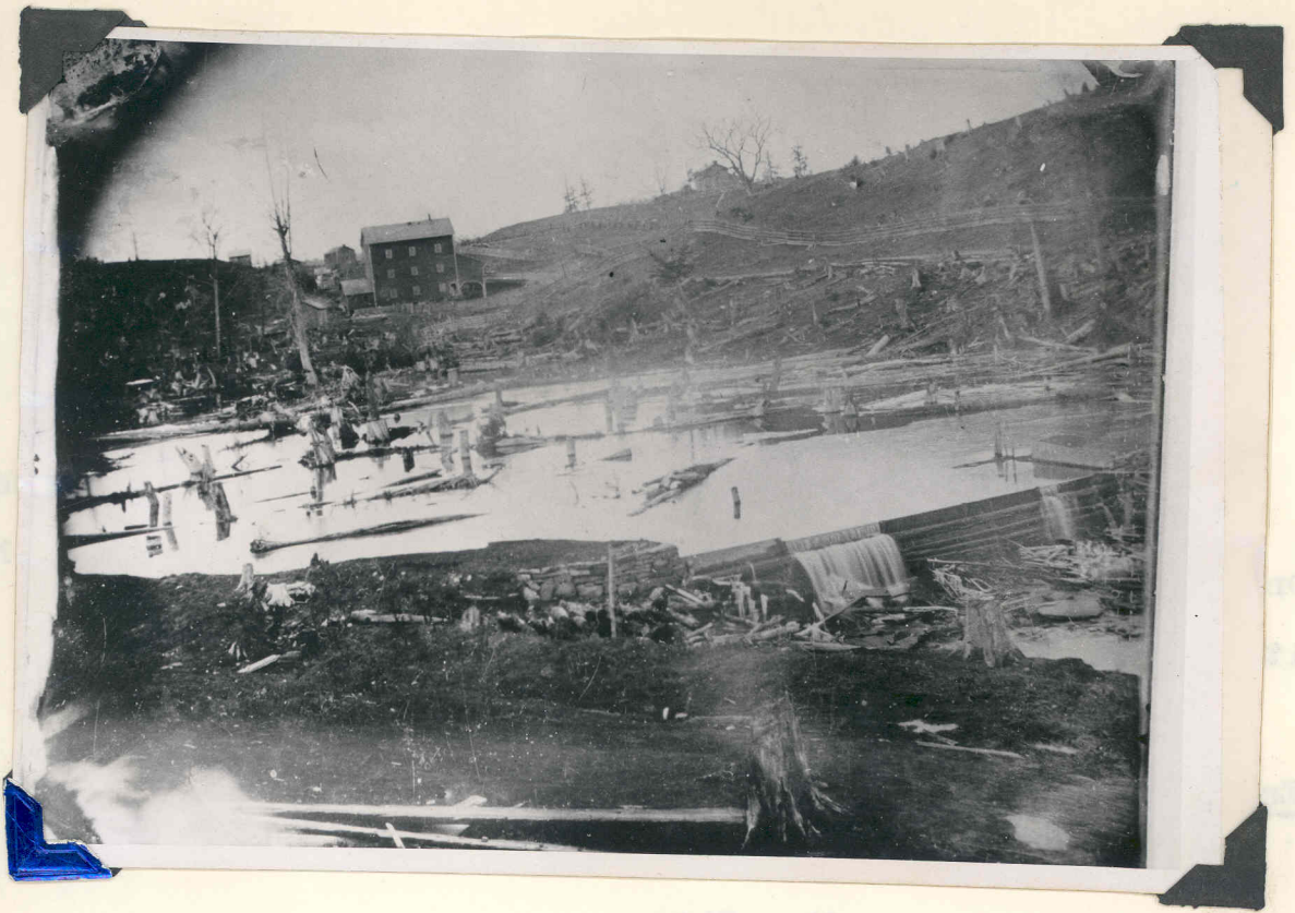
Picture of flour mill, built in 1849, situated on Baldwin farm on South side of lane, looking East.
