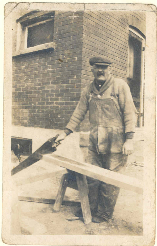
Ben Beynon building his house.
